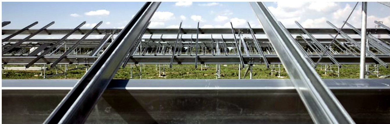
PV rails on C+ / Z rail beams · variant B
